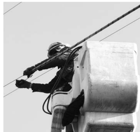
Left, turkeys at Gary Pratt's place now know to stay away from electric facilities. Photo courtesy of Gary Pratt. Right, KPUD lineman Martin Taylor wraps a colored guy guard around power lines so the birds can see the lines better as they fly to a nearby hillside. Photo by Andrew Christiansen of The Goldendale Sentinel.
