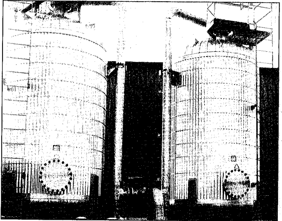
The tall tanks contain the carbon pellets media. The gas collected from the landfill will now filter through this gas-cleaning system before entering the engines at the landfill gas plant.
