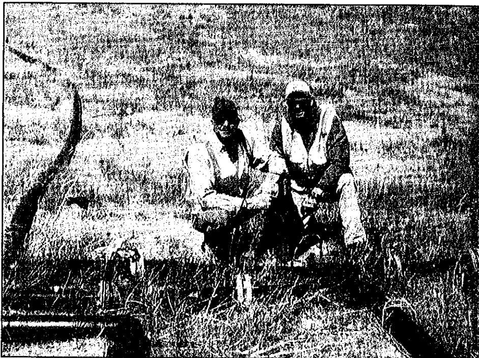
Jeff Link, left, regional disposal site technician, and Travis Gray, Klickitat PUD technician, inspect wellfield collection lines.
